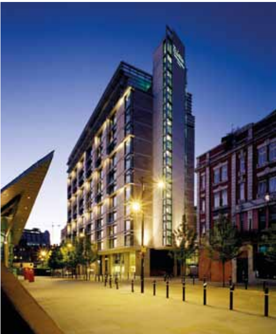
NORTHERN LIGHTS: Laing O'Rourke's UK refurbishment projects in the north include the conversion of Manchester's debating and concert venue Free Trade Hall into a Radisson Edwardian hotel (left), and Sheffield's Meadowhall shopping centre (below)
