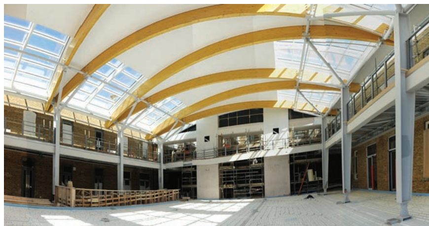
Opposite LUSU during refurbishment Top: The Square Above: The Square under construction
