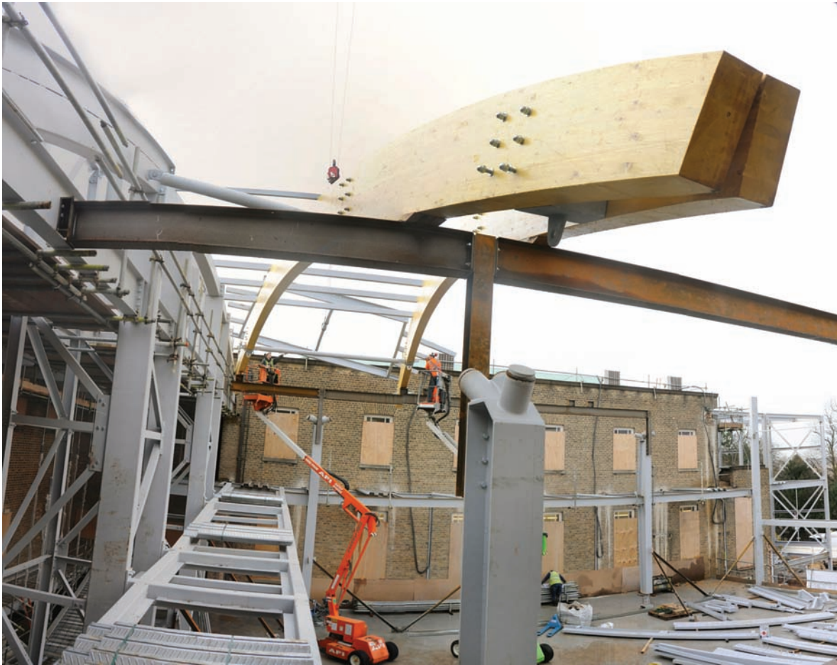
The roof under construction
